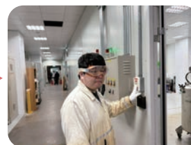
Activation of emergency exhaust ventilation system
