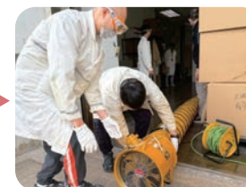
Installation of portable fans for fresh air circulation
